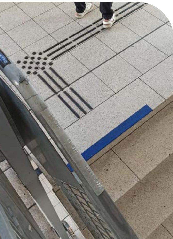
Image 3 | A tactile wayfinding surface indicating a change in level at Volksparkstadion Hamburg
