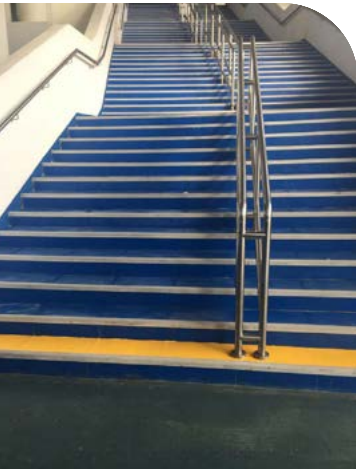
Image 14 | A stairway with uniform steps, handrails and contrasting step edges at Fisht Olympic Stadium, Sochi
