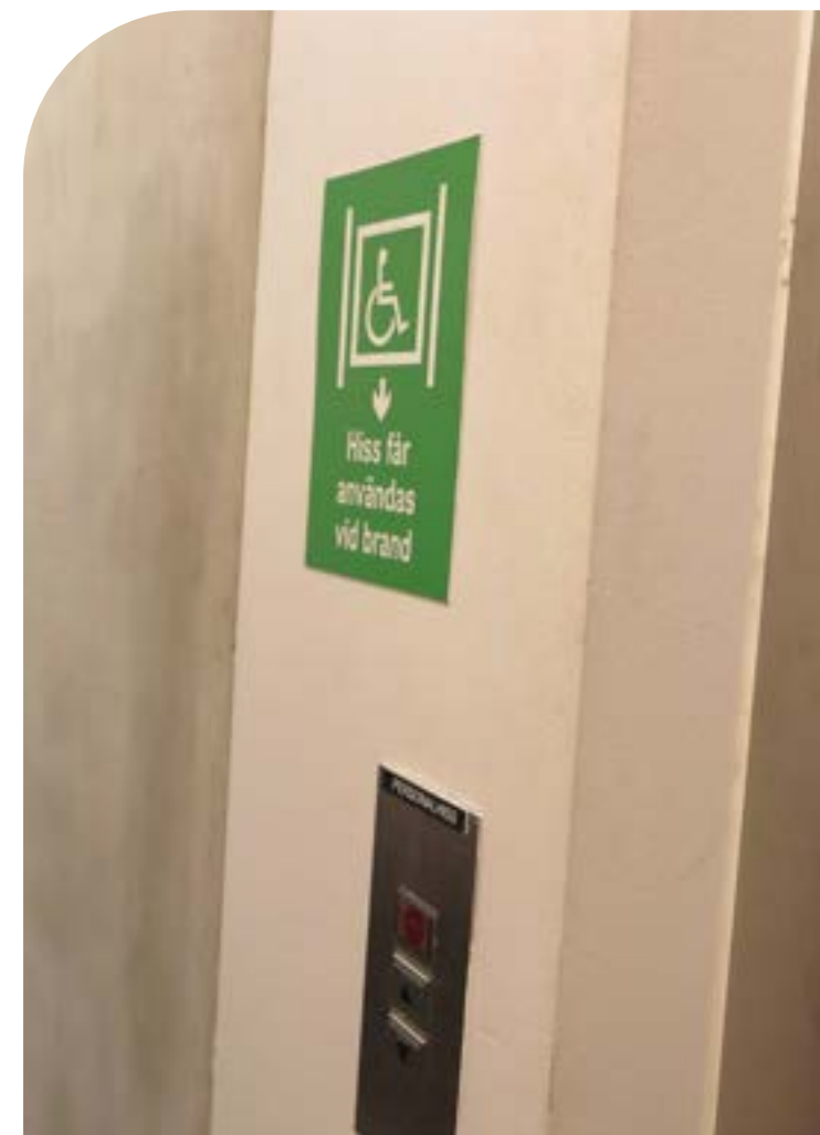
Image 24 | Evacuation lift sign at Sweden's Nationalarenan
