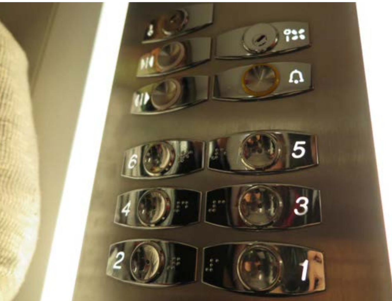
Image 10 | A lift control panel with tactile and Braille symbols at the National Stadium of Wales
